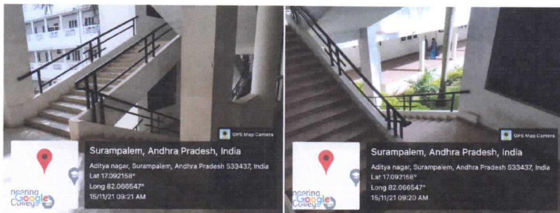
Hand Railed Stair Case
