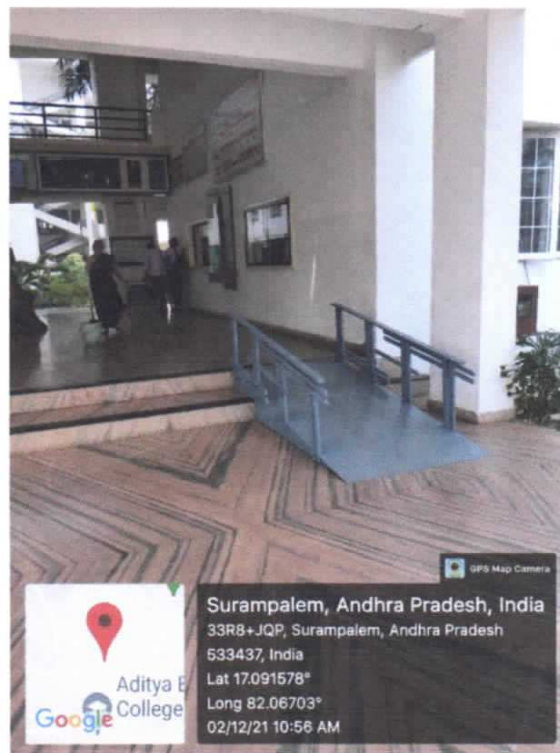
Disable Friendly Ramp At C.V.Raman Block Aditya College Of Engineering & Technology
